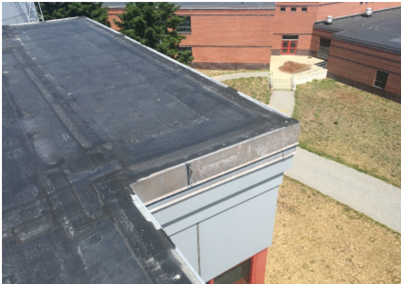
Photo C3 - Metal Gravel Stop
