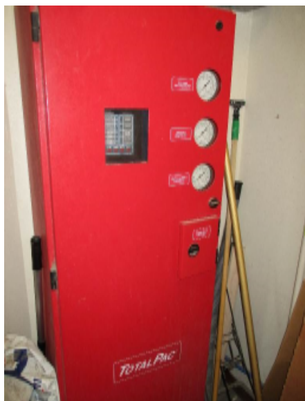
Photo H5 - Abandoned Pre-Action System at High School
