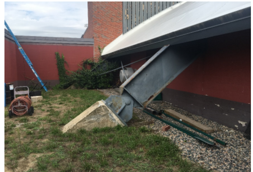
Photo C12 - Steel Arch Base
