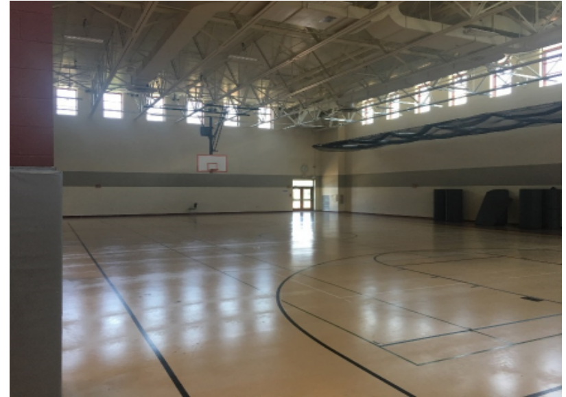
Photo D2 - Acoustical Metal Deck
