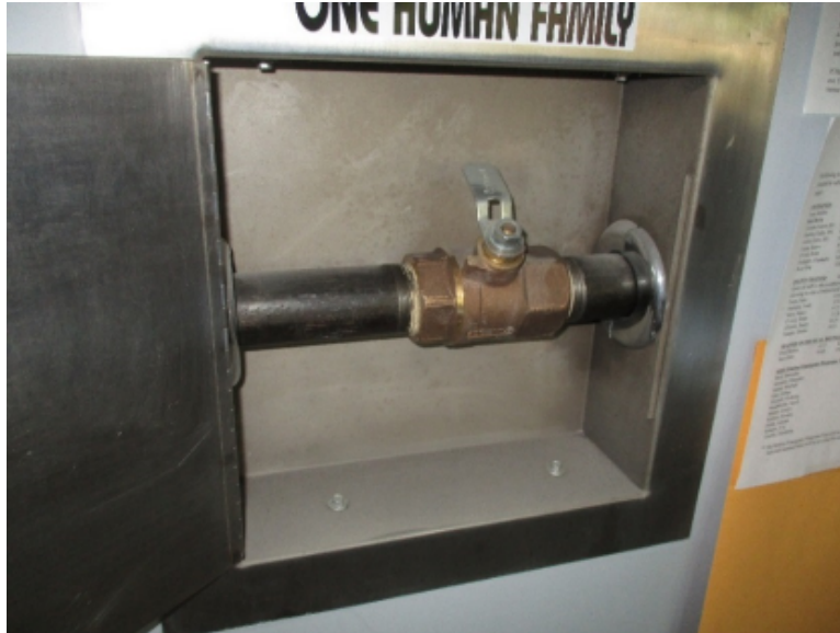
Photo H33 - Gas Service - Shutoff at Science CR
