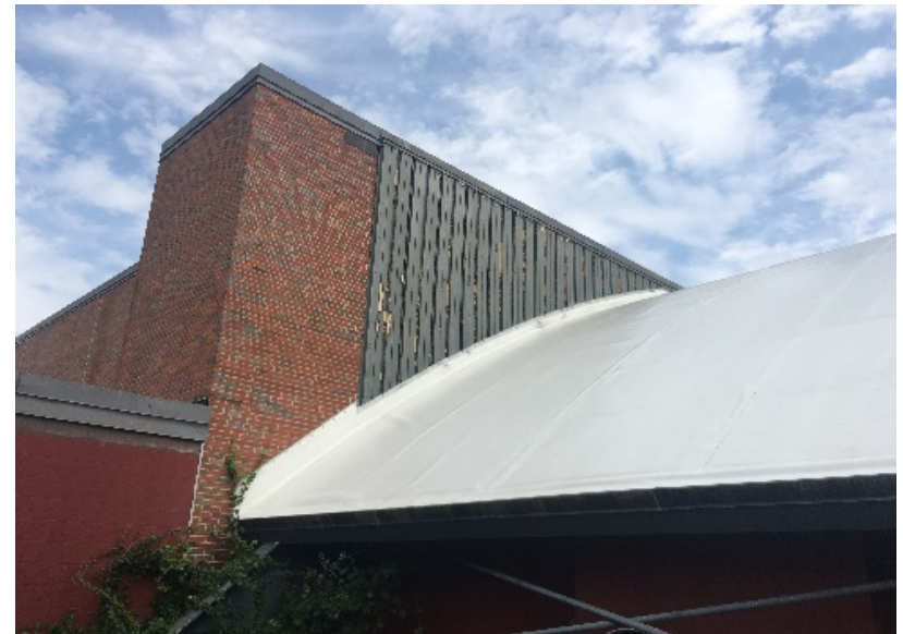
Photo C4 - PVC Roof
