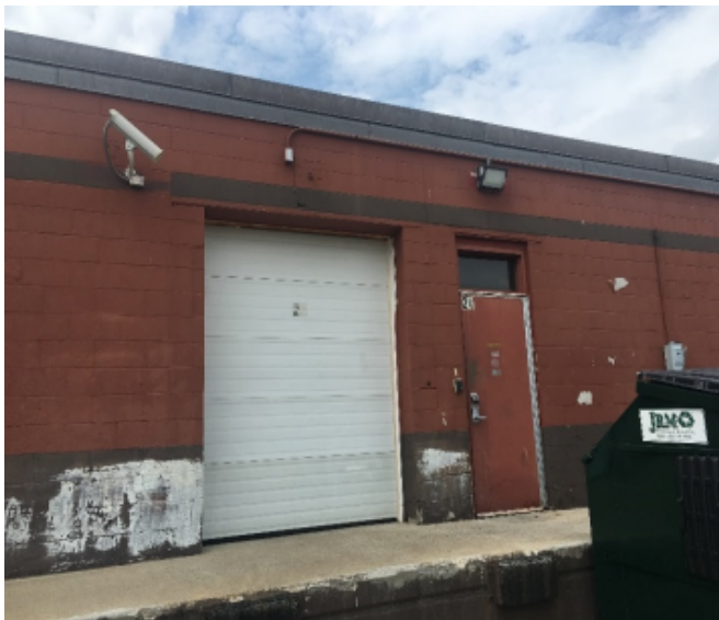
Photo C11 - Exterior Overhead and Hollow Metal Doors
