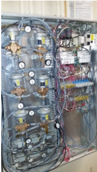
Photo G16 - Automatic Temperature Controls
