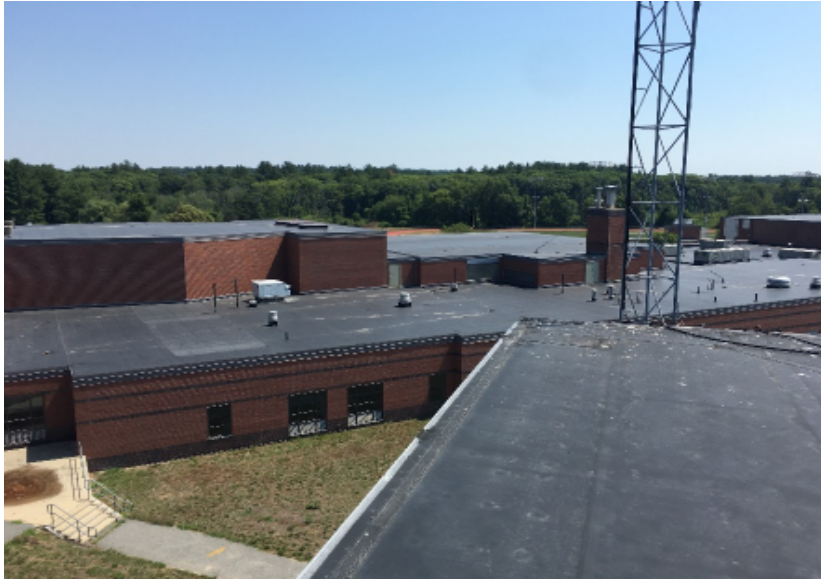
Photo C1 - EDPM Roof
