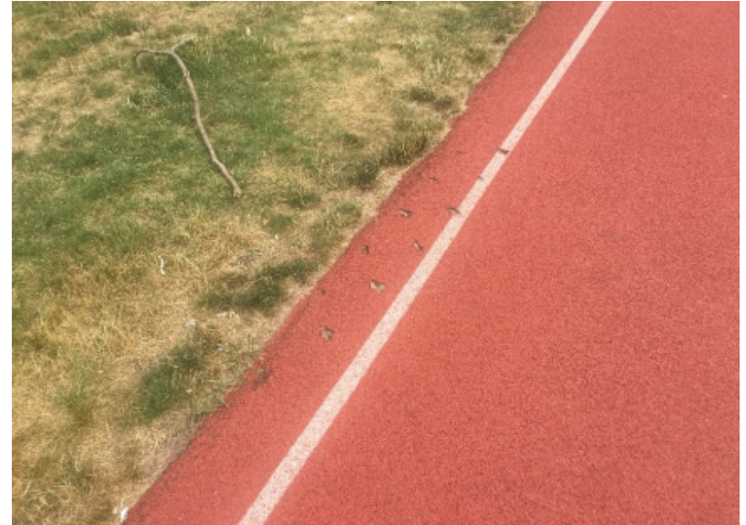
Photo B2 - Track surface damage
