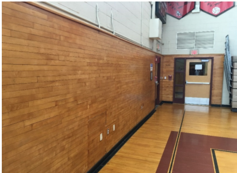
Photo D7 - Wood Strip Cladding
