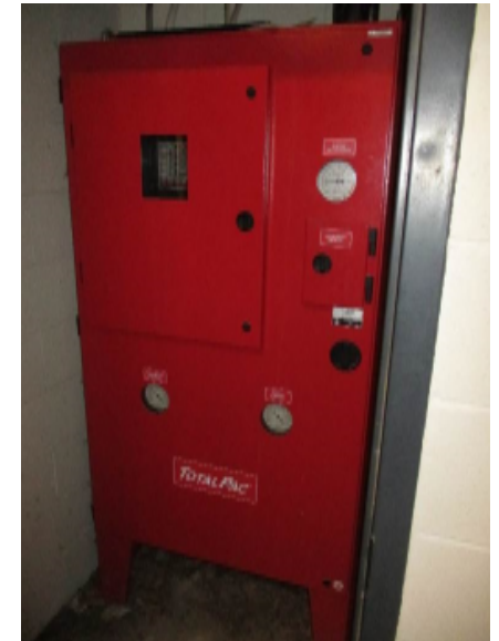
Photo H4 - Wastewater Treatment Building Pre-Action System
