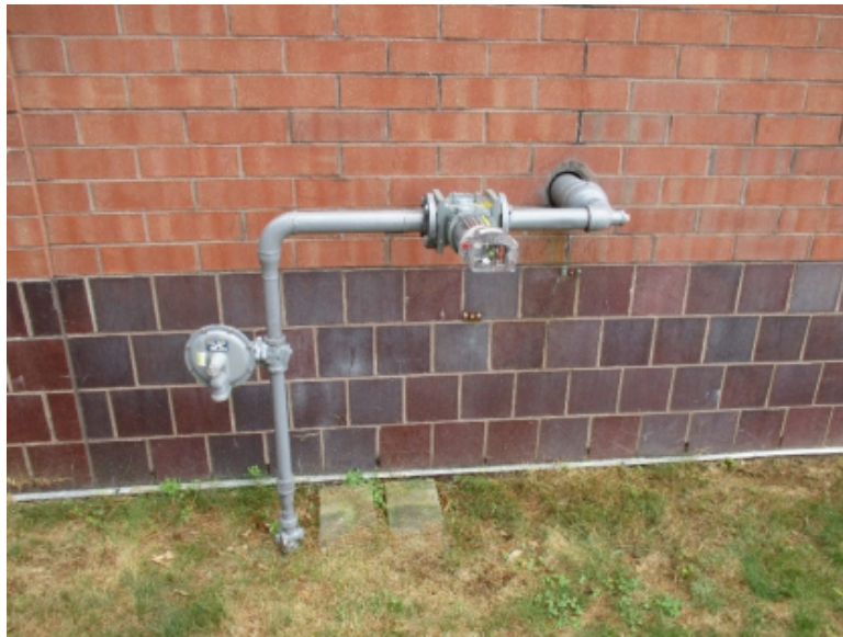
Photo H35 - Waste Water Treatment Gas Service
