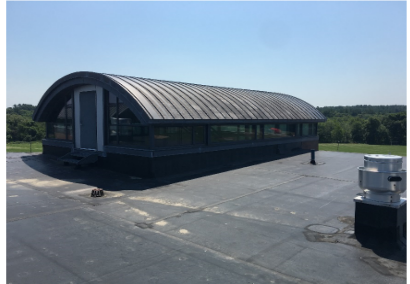
Photo C2 - Lead Coated Copper (Metal) Roofing
