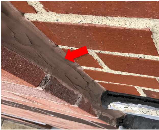
Figure 35: View of failed expansion joint sealant.
