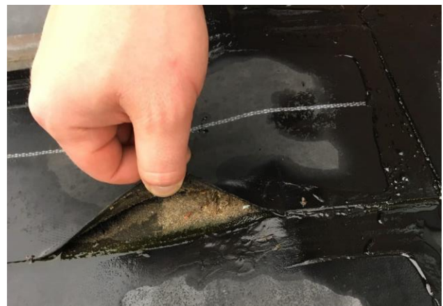
Figure 12: Delaminated roof membrane patch observed on Roof Area B.2.
