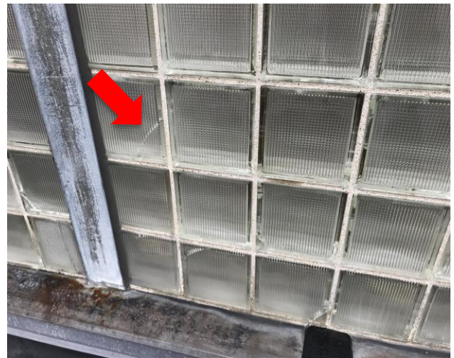
Figure 32: View of cracked glass block.
