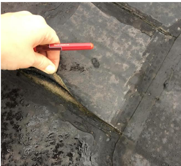
Figure 13: Delaminated roof membrane patch observed on Roof Area A.
