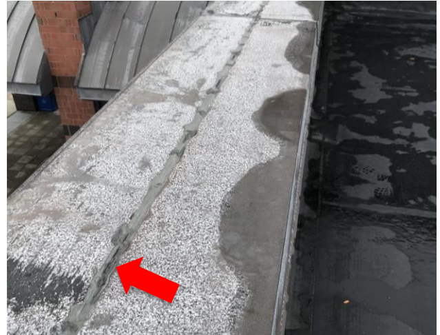
Figure 20: Failed seams observed in two-piece parapet cap flashing on Roof Area B.2.
