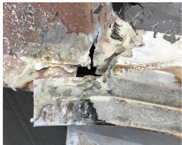
Figure 16: View of cracked solder and open sheet metal flashing seams at a scupper on Roof Area B.3.
