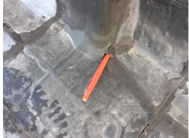
Figure 10: Open area of roof membrane were observed.
