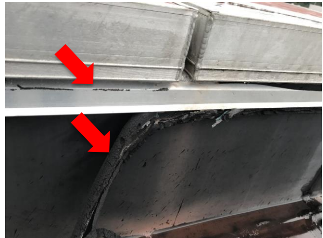
Figure 41: View of smoke hatch with failed weatherstripping and missing sealant.
