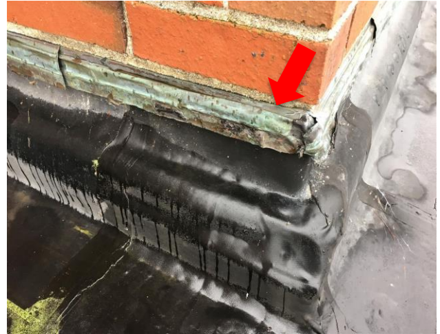
Figure 31: View of throughwall flashing with open joints.
