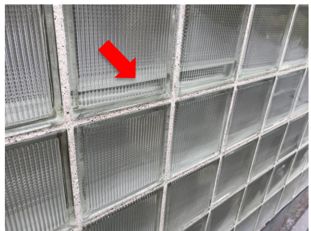
Figure 33: View of glass block filled with water.
