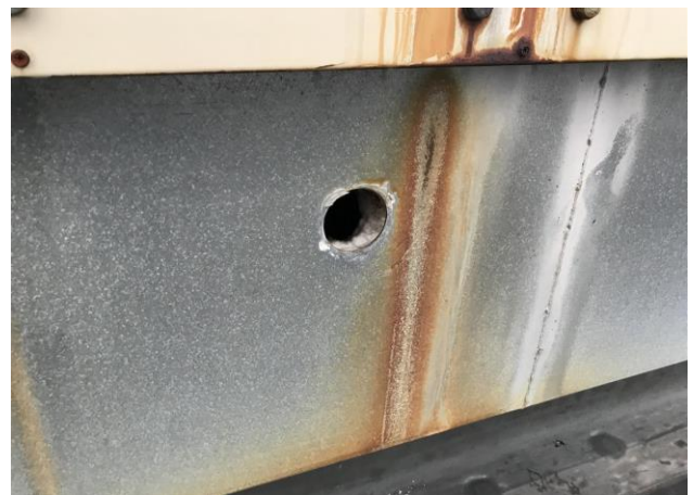
Figure 39: Open penetrations in RTU curbs.
