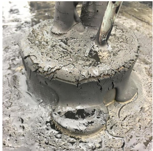
Figure 15: Failed sealant at the pitch pockets observed.
