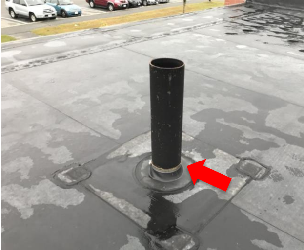
Figure 17: Low flashing height observed at a vent pipe on Roof Area B.
