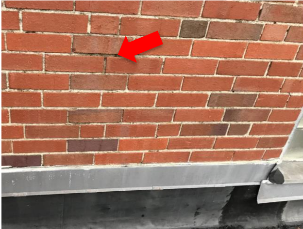
Figure 34: View of deteriorated mortar.
