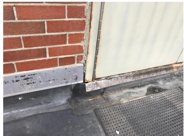
Figure 27: Scope 4 area close up view of the poor door pan flashing.
