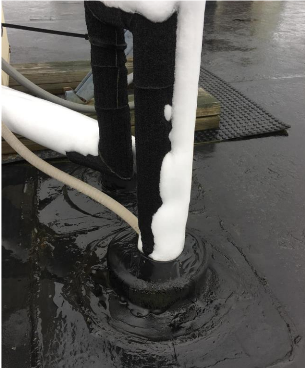
Figure 40: View of frozen air conditioner lines on Roof Area A.
