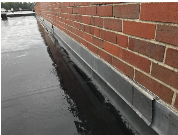
Figure 30: Failed sealants were typically observed at reglet joints.
