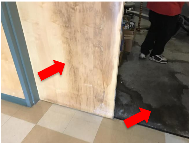
Figure 2: Water staining observed on door and floor of Mechanical Room H331.
