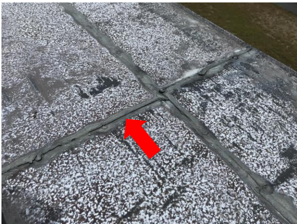
Figure 19: Failed seams observed in two-piece parapet cap flashing on Roof Area B.2.
