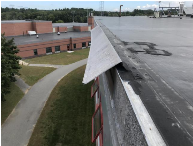
Figure 18: Displaced edge metal observed on Roof Area A.
