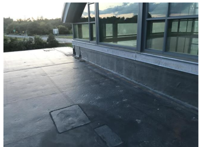
Figure 24: Scope 2 area active leak on rising wall on Roof Area A
