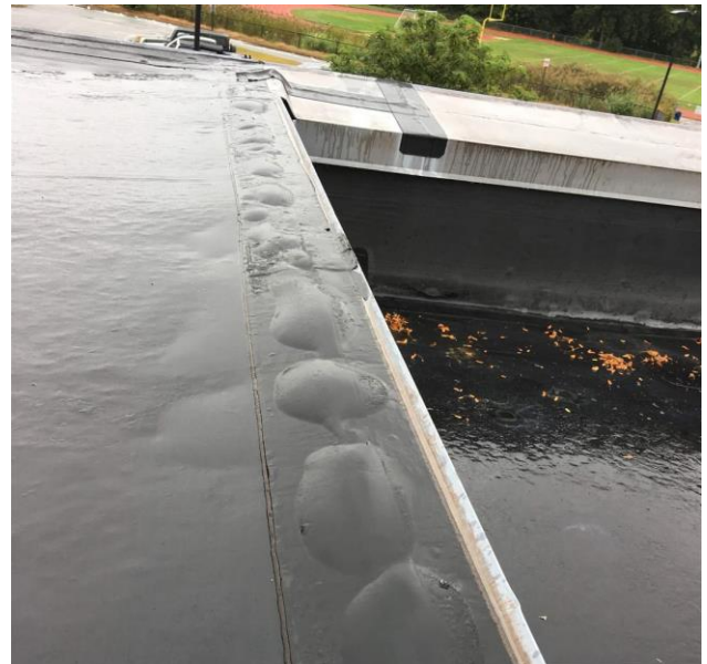
Figure 21: View of bubbled stripping membrane at edge of Roof Area C.1.
