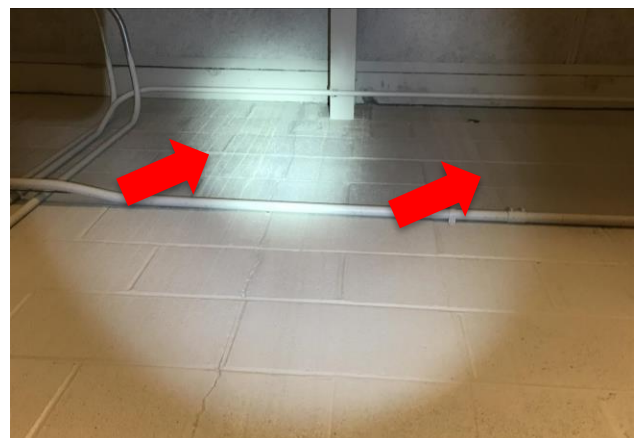
Figure 4: Water staining observed along rising wall of Corridor EC108.
