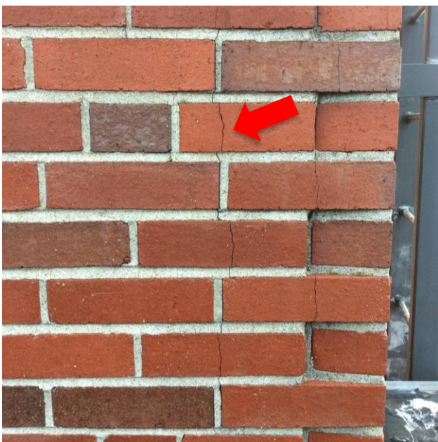
Figure 36: View of step cracking.
