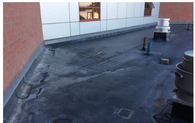
Figure 22: Scope 1 area, wet insulation and unadhered membrane was observed.
