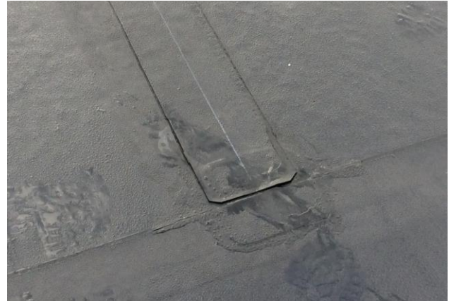
Figure 14: Delaminated stripping membrane observed on Roof Area F.3.
