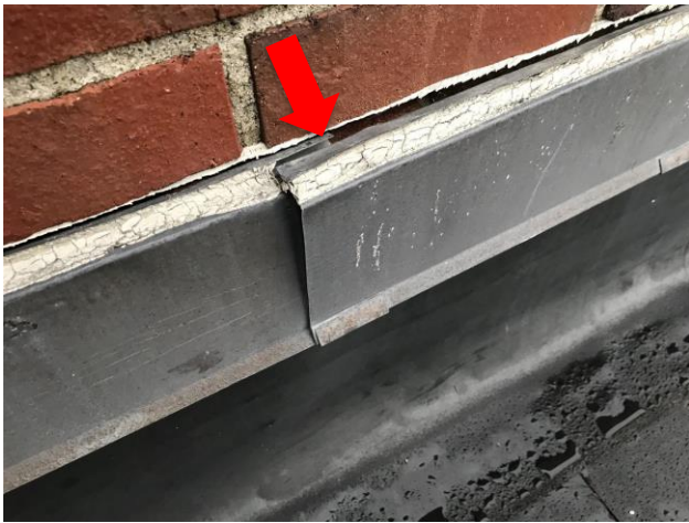
Figure 29: Reglet joint observed pulled out of wall and open.
