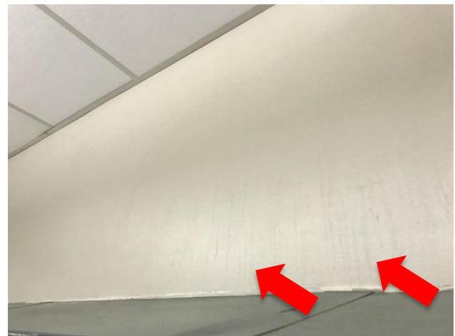
Figure 1: Water staining observed above lockers in Corridor HC301.
