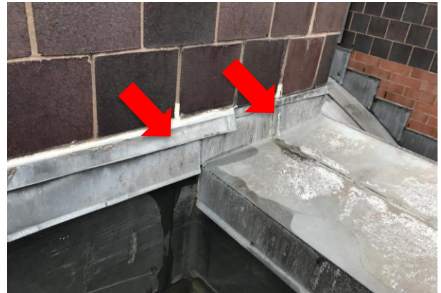
Figure 38: View of masonry weeps filled with spray foam.
