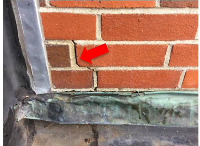
Figure 37: View of step cracking.
