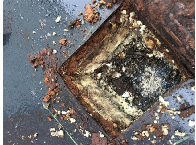
Figure 44: View of wet roofing material.
