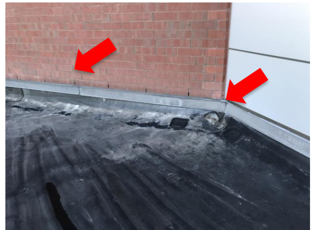
Figure 23: Scope 1 area, throughwall flashing joint in the corner appears to be open.
