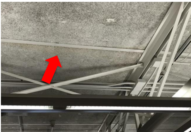
Figure 3: Stained roof deck observed in Cafeteria C106.
