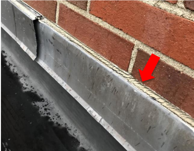
Figure 28: Failed sealant observed at reglet joint flashing terminations on the rising wall of Roof Area B.3.
