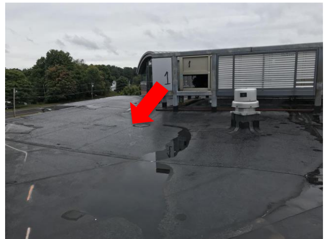
Figure 11: View of unadhered membrane on Roof Area A.
